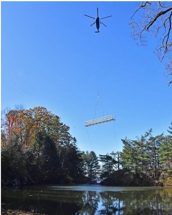
Figure 4.9: A prefabricated bridge transported by helicopter
