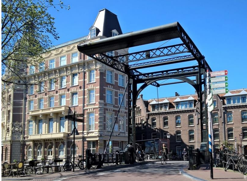
Figure 4.11: Aluminium bridge with maintenance-free movable deck, Amsterdam (the Netherlands)
